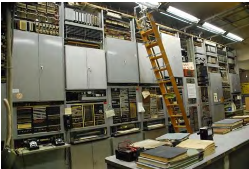
Figure 8. C&P Number 5 Crossbar Switch
